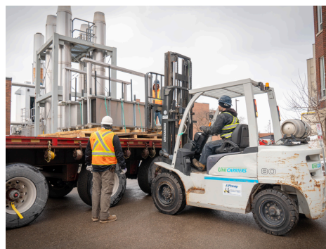
Two new heat exchanger units arrive at BGH, a crucial part of the upgraded cooling system for the new air handling unit.
